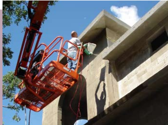
Microscopic, needle-like crystals fill the naturally occurring pores and capillary tracts of concrete for guaranteed waterproof structures.
